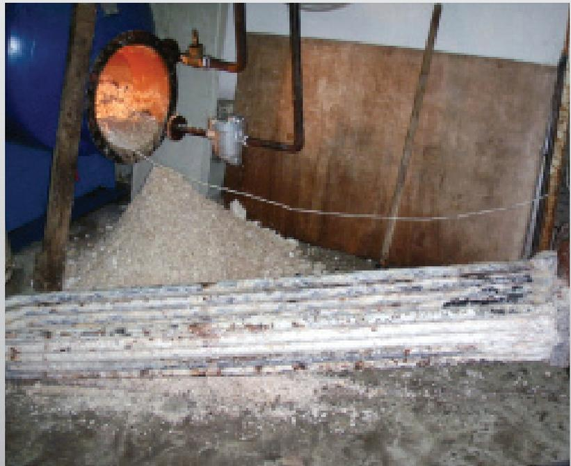
Figure : Water Heater with a Heat Exchanger heated by steam
